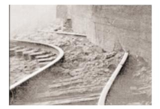
Figure 3. Bent rails inside the Kern County urban railway tunnel. The White Wolf Fault had a both compressive and lateral dislocation during the 1952 Kern County earthquake. Indicative of this type of fault dislocation is the fact that the rails are bent and continuous underneath the tunnel wall, showing that the wall was lifted up enough for the rail to slide underneath. Source: SCECDC 2002.
