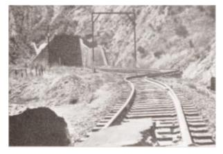
Figure 2. Kern County urban railway tunnel. A view from the entrance of the tunnel showing bent rails near a zone of intense fracturing along the White Wolf Fault. Source: SCECDC 2002.
