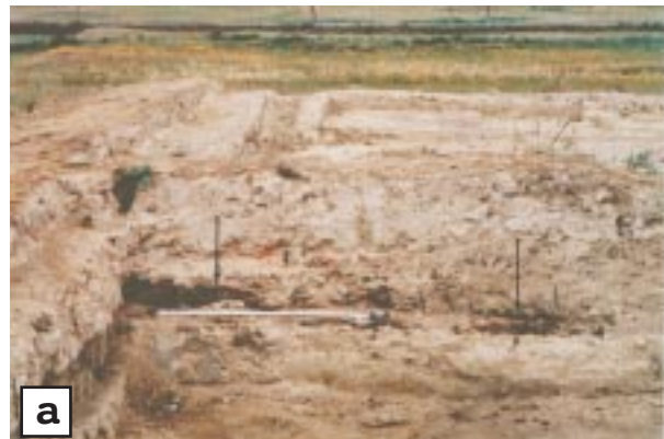
Figure 8. Shift and tilt in a northeast direction of lower course of masonry of saman bricks in room No. 16. Angle of declination of deformed wall is between the solid line (modern wall inclination) and the dashed line (originally vertical wall).
