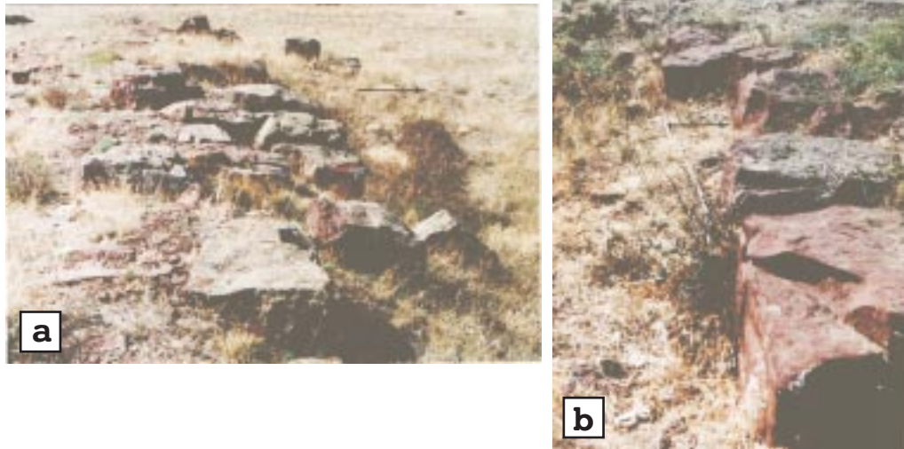
Figure 20. Northward shift of stone blocks (shown by arrows) of northern city wall: (a) to the north from rooms No. 2 and 3, dashed line shows original position of the stones; (b) southern wall of room No. 1.
