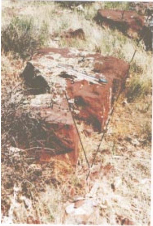
Figure 21. Counter-clockwise rotation of a stone block measuring 75x50x40 cm. Blocks 1–3 were preserved in their original positions. Block 4 was rotated.
