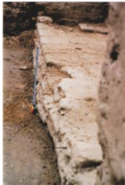
Figure 13. Shift of a lower course of bricks in a step at the temple entrance.
