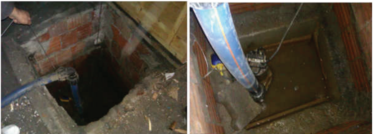
Figure 10. Pictures of drill hole in the basement of the Police Department, located 15 m away from point KH07 (40°18'05"N, 37°49'26"E).
