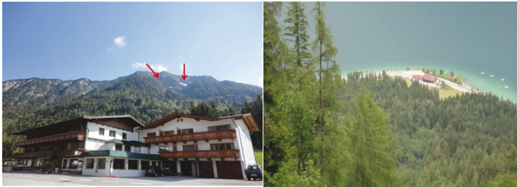
Figure 3. Overview of the endangered hotel.
