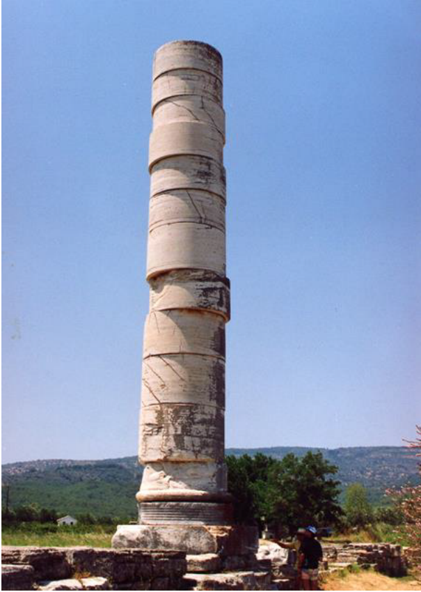
Figure 6. Offsets between drums are clear in the only surviving column of the Heraion Temple in Samos (for location see Figure 1) and originate from oscillations (rocking) during strong earthquakes, as explained in Figure 5.
