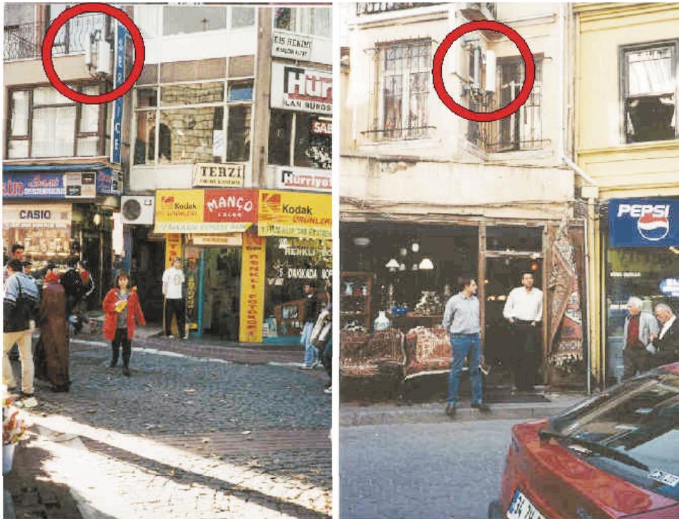
Figure 1. Two base station antenna locations in Kadıköy (in Istanbul). Measured electric field strength on the ground varies between 2 V/m and 6 V/m.
