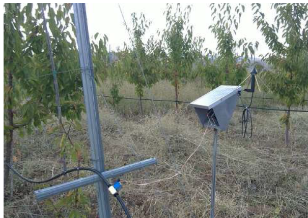
Figure 10. View of installed electrovalve unit.
