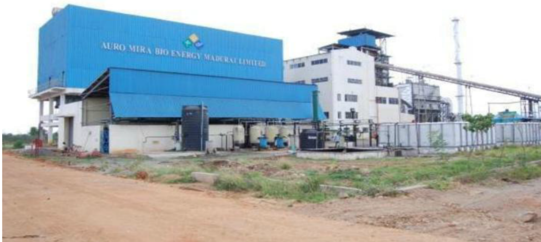
Figure 1. Front view of the grid connected biomass plant.
