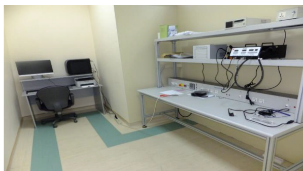
Figure 15. Measurement laboratory next to the test cell separated by a cable canal only.
