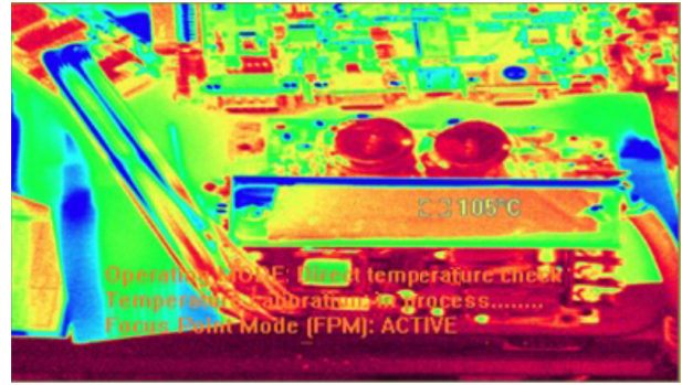
Figure 25. Thermal camera screen capture for IGBT module skin temperature test.
