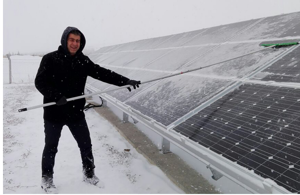
Figure 2. Snow clearing activity of array with a squeegee.
