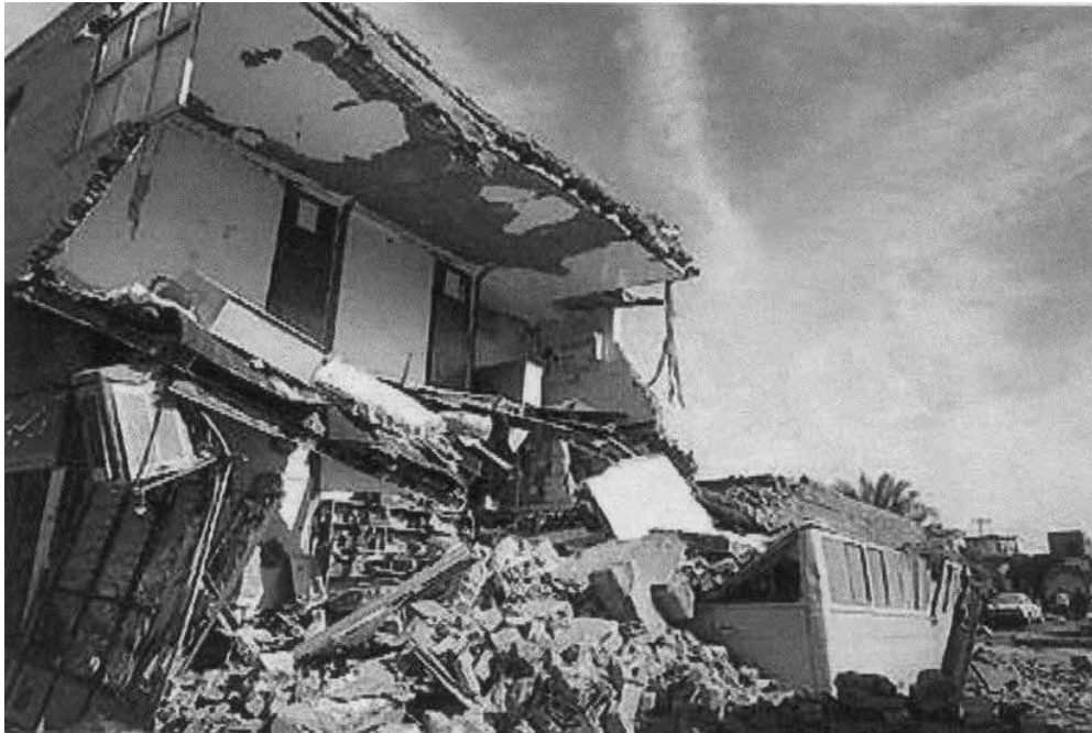
Figure 5. Out-of-plane failure of a 2nd story wall in the Bam Earthquake, 2003.
