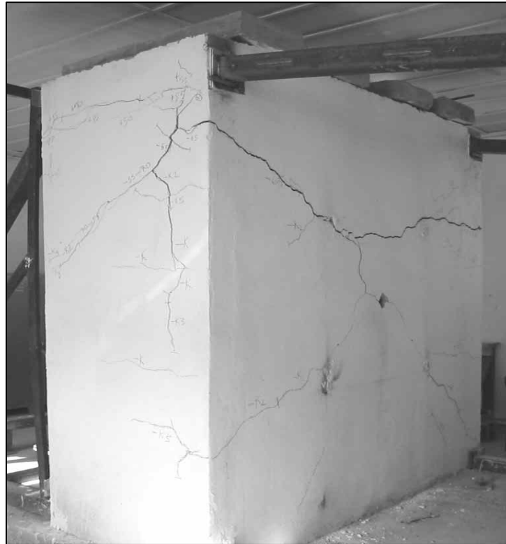
Figure 13. Cracking pattern of the test wall at failure.
