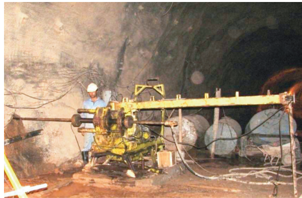
Figure 3. Drilling machine (SD300) while drilling horizontal borehole.
